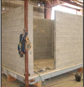
concrete block walls
